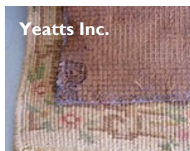
Deteriorating underlay
